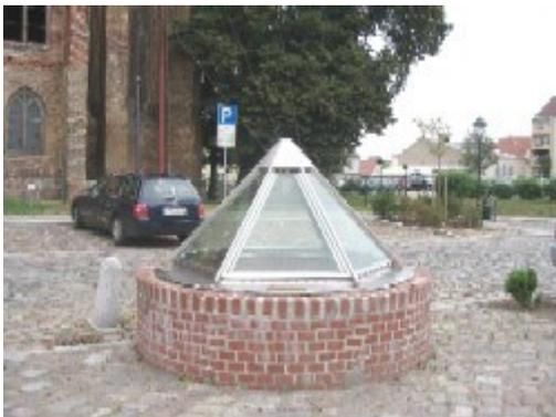
The well was rediscovered during roadwork in 2001 and promptly restored. It still served in 1900 to supply drinking water. It has a depth of 7 meters and a diameter of 1.60 m.
